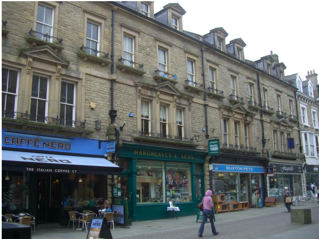
Nos. 12 to 28 Spring Gardens Row of six shops built during the 1860's
