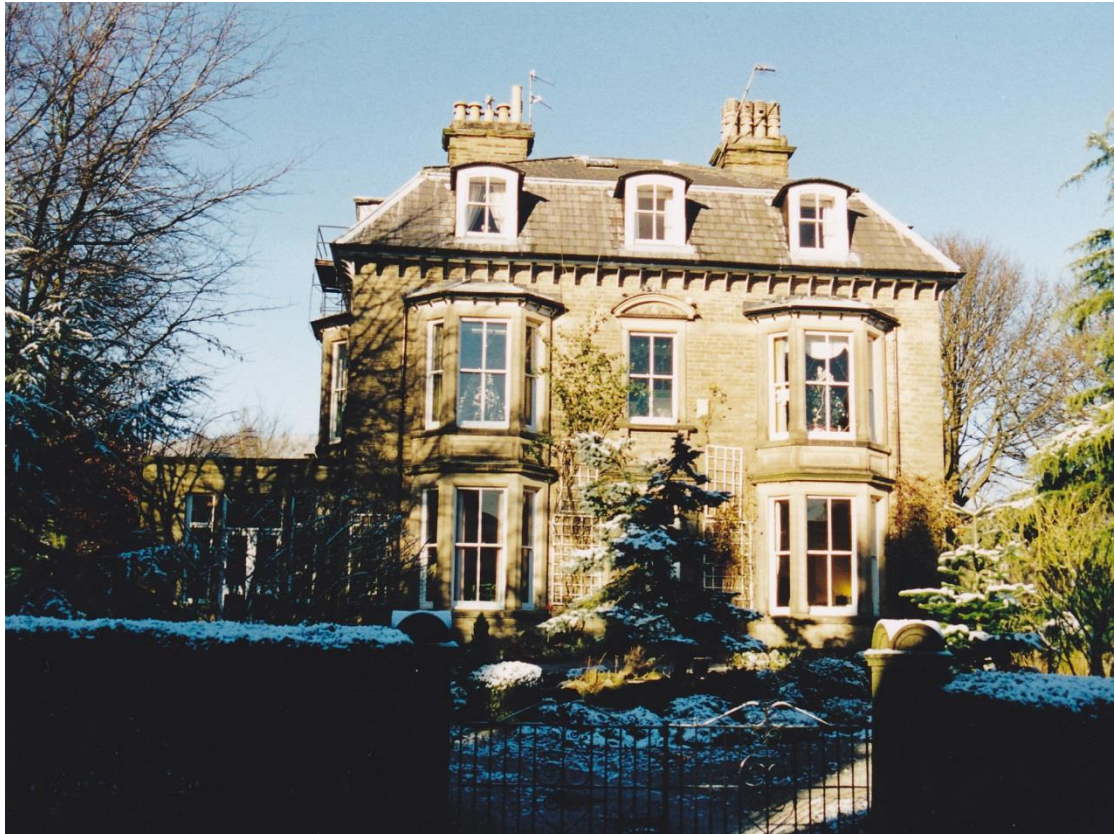
Claremont No 20 St. John's Road Built 1876
