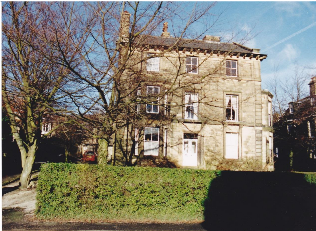
Cranford No 22 St. John's Road Formerly Cumbermere House built c1800
