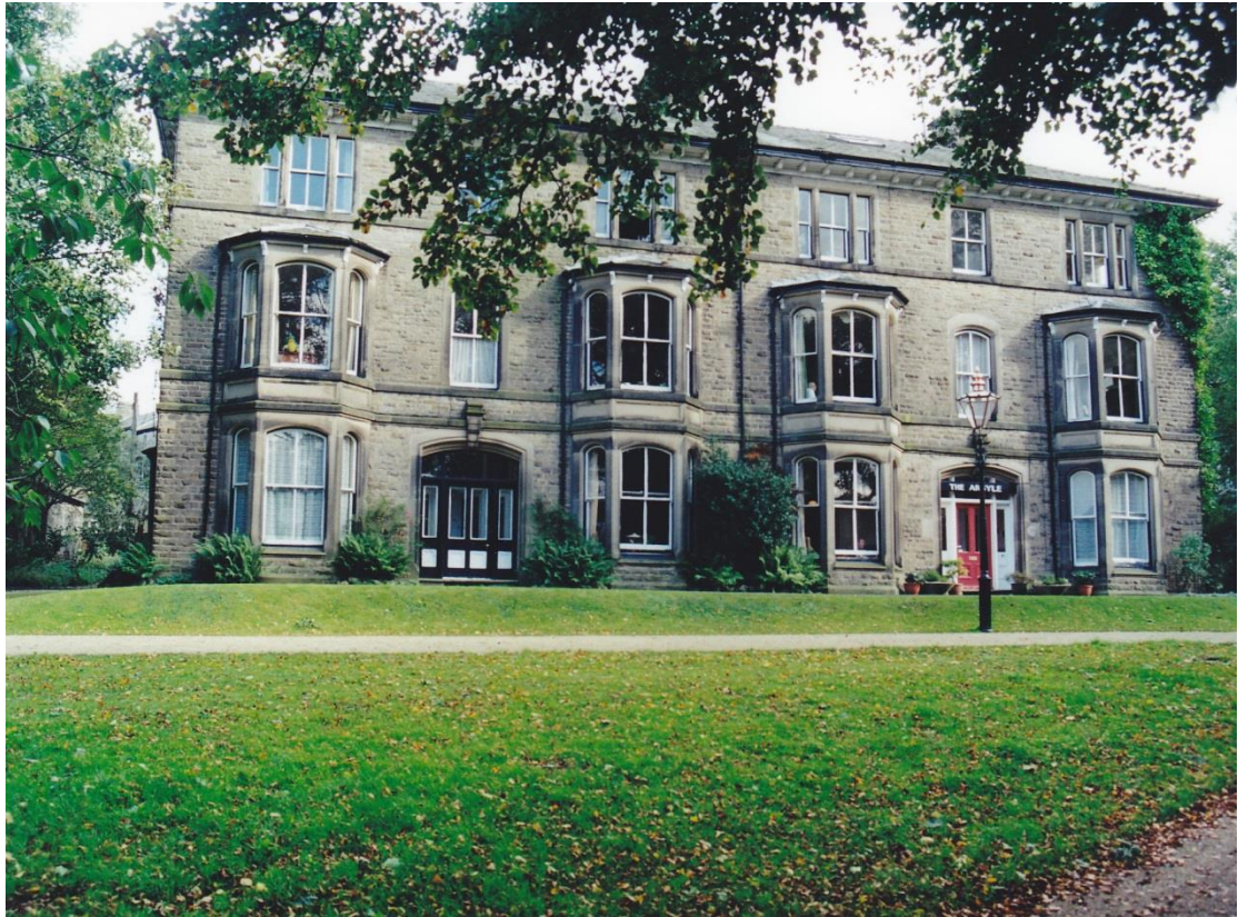
Nos 24-25 Argyle Villas, built 1875-76 for E C Milligan, local draper. Architect – probably Robert Rippon Duke.
