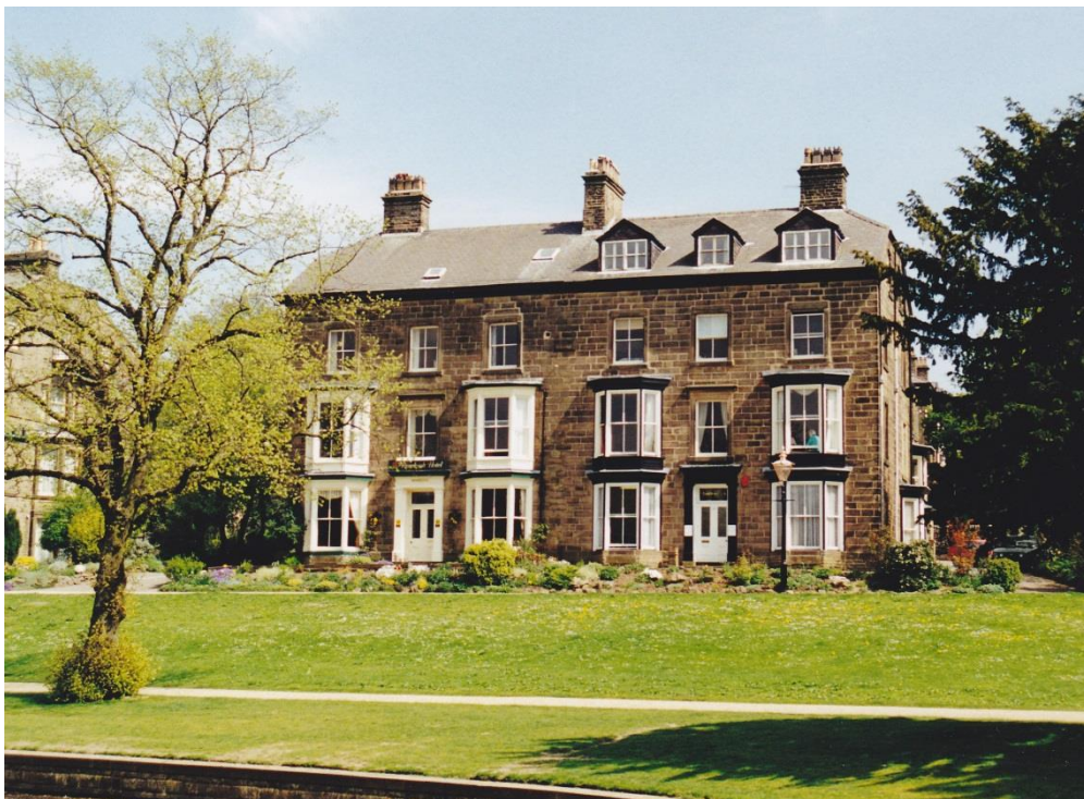
No 19 (Roseleigh Hotel) and No 20 (The Sherwood) Formerly Cambridge Villas c1867-68.
